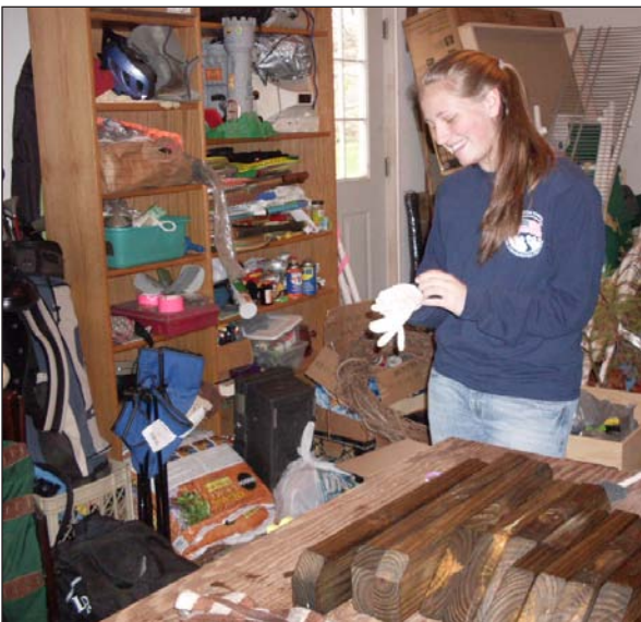
Katie applying finish to the framing.
